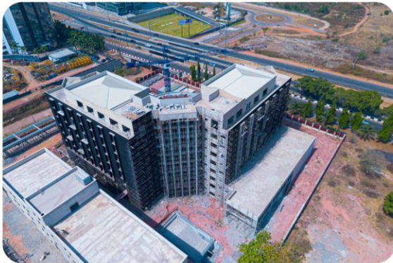
CONSTRUCTION OF JOHN WILLIAMS HOTELS AND RESORTS LIMITED, ABUJA
